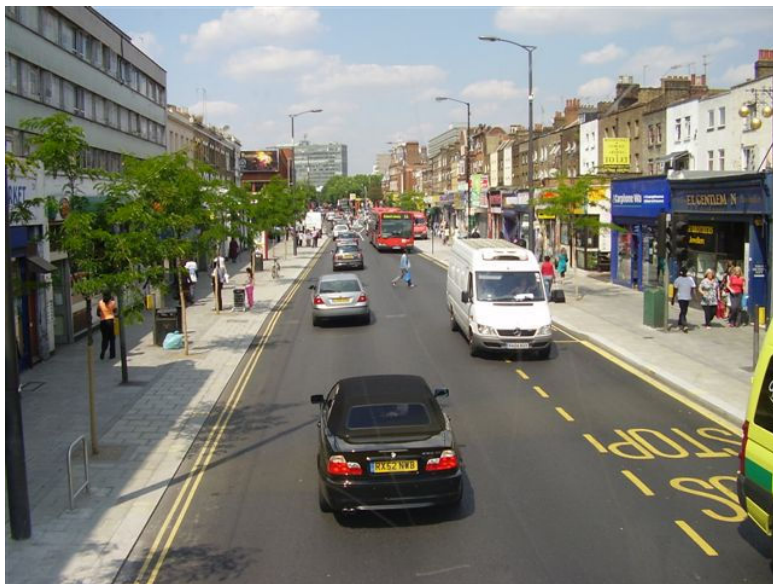
Walworth Road – 17,600 vehicles per day
